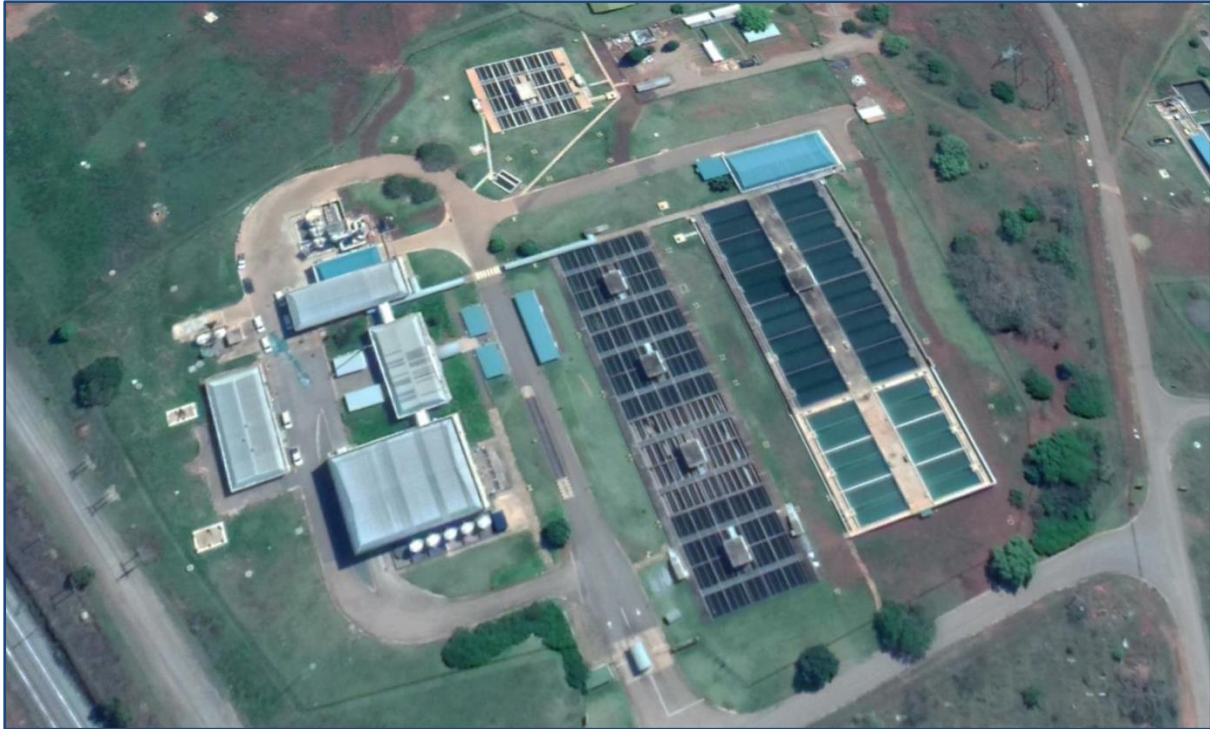
Figure 7.29 Midmar Water Treatment Plant after the upgrade.
