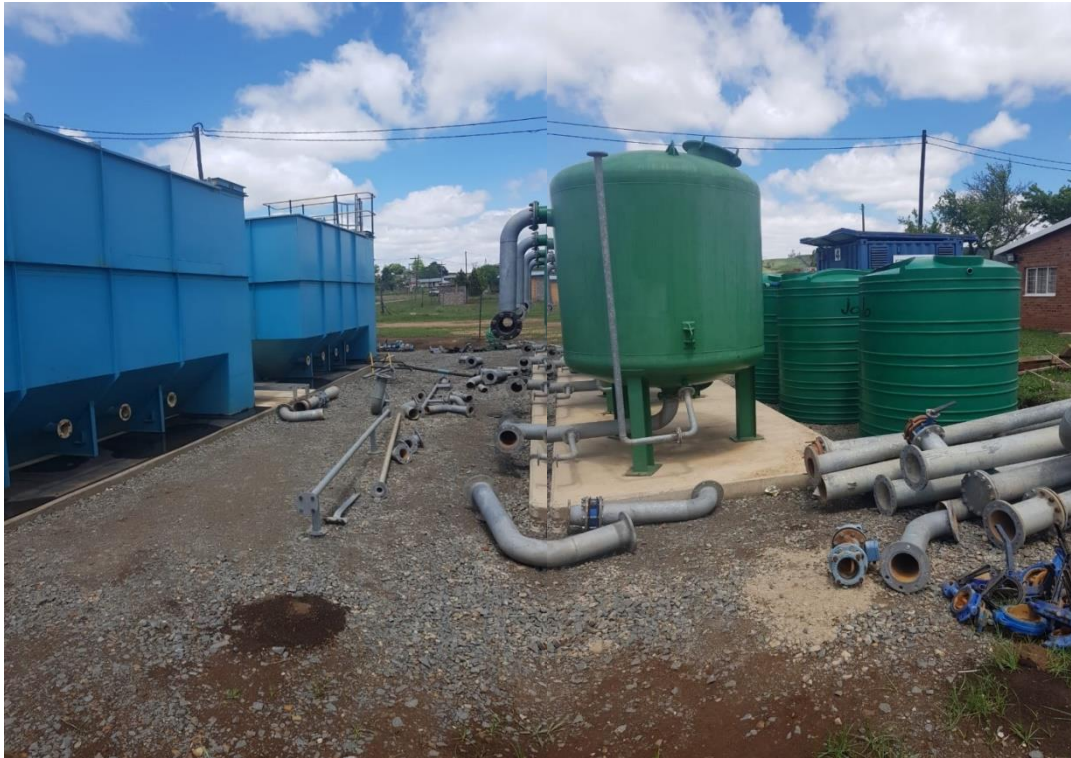
Figure 7.73 1 MI/day being constructed at the Lidgetton System.
