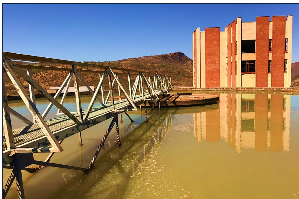
Figure 13.24 Ezakheni Water Treatment Plant (unknown date).
