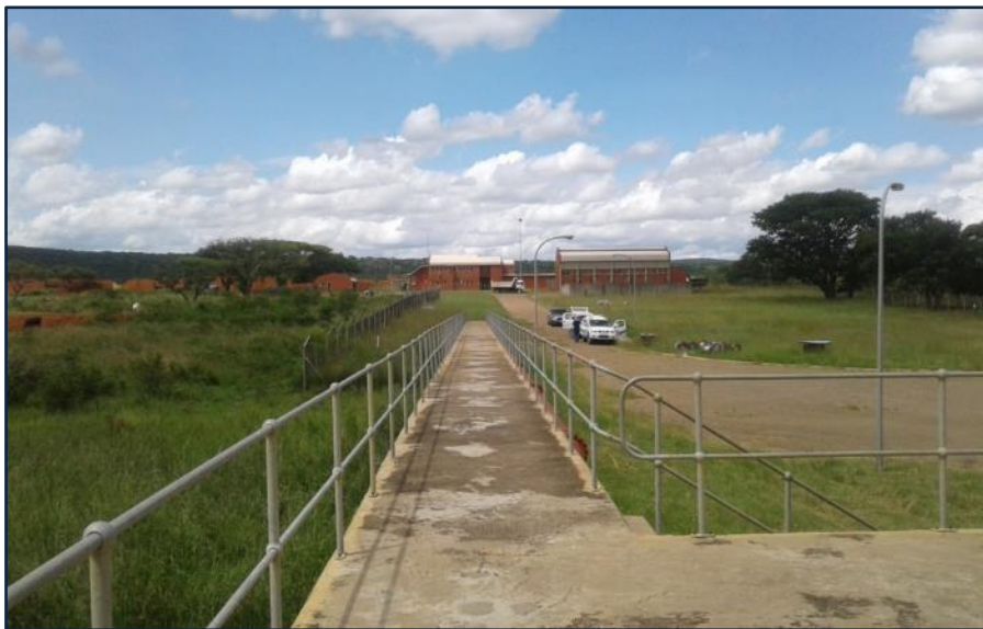
Figure 13.38 Olifantskop Water Treatment Plant (unknown date).
