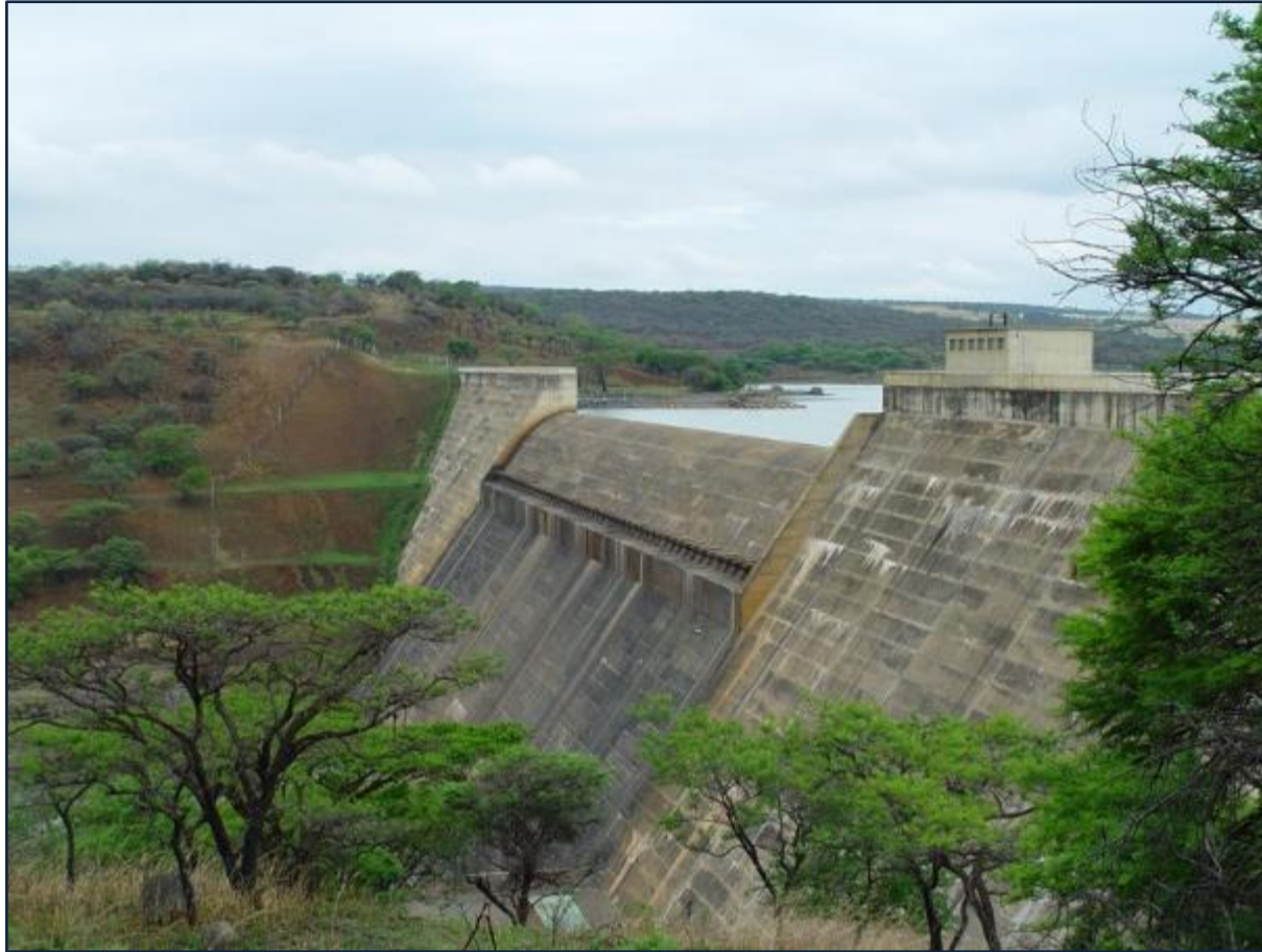
Figure 13.20 Spioenkop Dam (DWS unknown date: DWS website).
