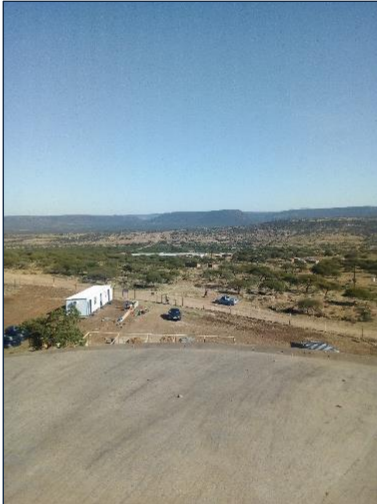
Figure 13.44 Pipeline servitude from Petronella Reservoir (Umgeni Water 2019).
