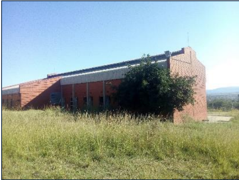
Figure 13.45 Petronella Reservoir Pump Station (Umgeni Water 2019).
