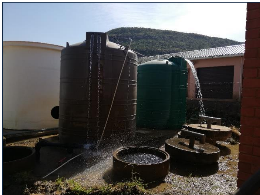
Figure 13.34 Tugela Estates WTP reservoirs (Umgeni Water 2019).
