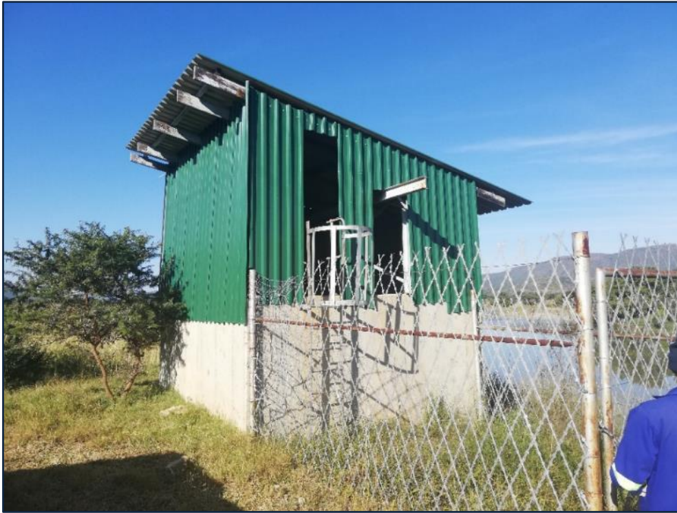
Figure 13.31 Tugela Estates Raw Water Pump Station (Umgeni Water 2019).
