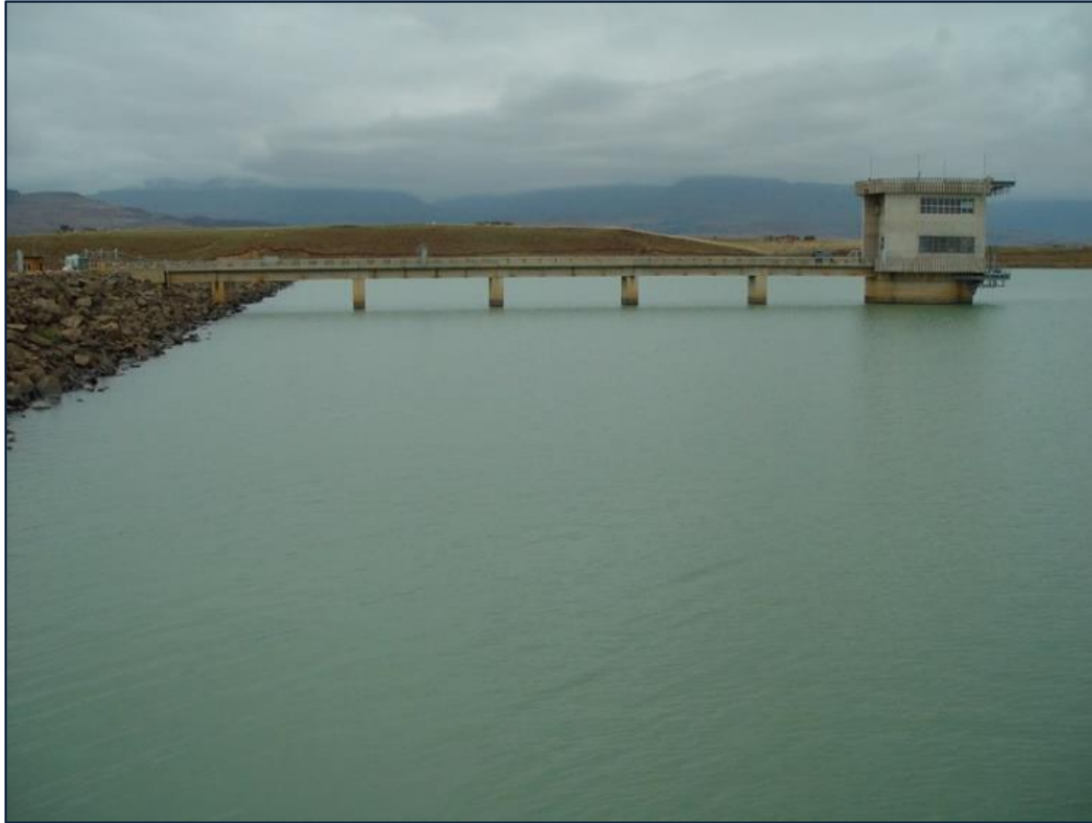
Figure 13.17 Woodstock Dam (DWS unknown date: DWS website).
