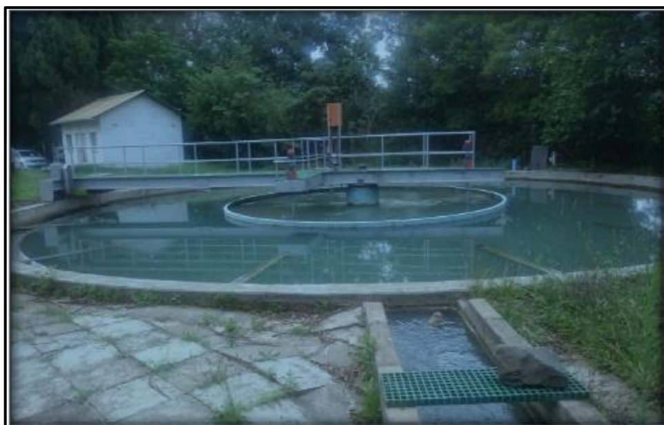
Figure 13.61 Archie Rodel WTP (Umgeni Water 2017)
