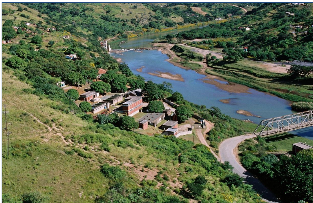
Figure 11.27 Craigieburn Water Treatment Plant (decommissioned).
