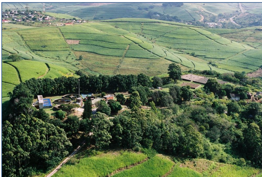
Figure 11.28 Umzinto Water Treatment Plant.
