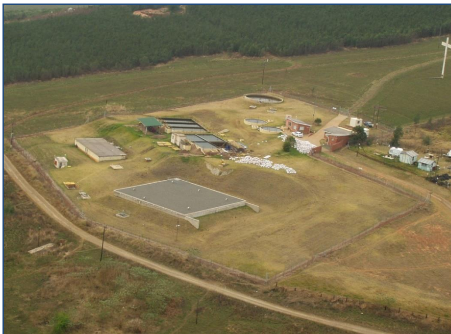
Figure 8.5 Ixopo Water Treatment Plant.
