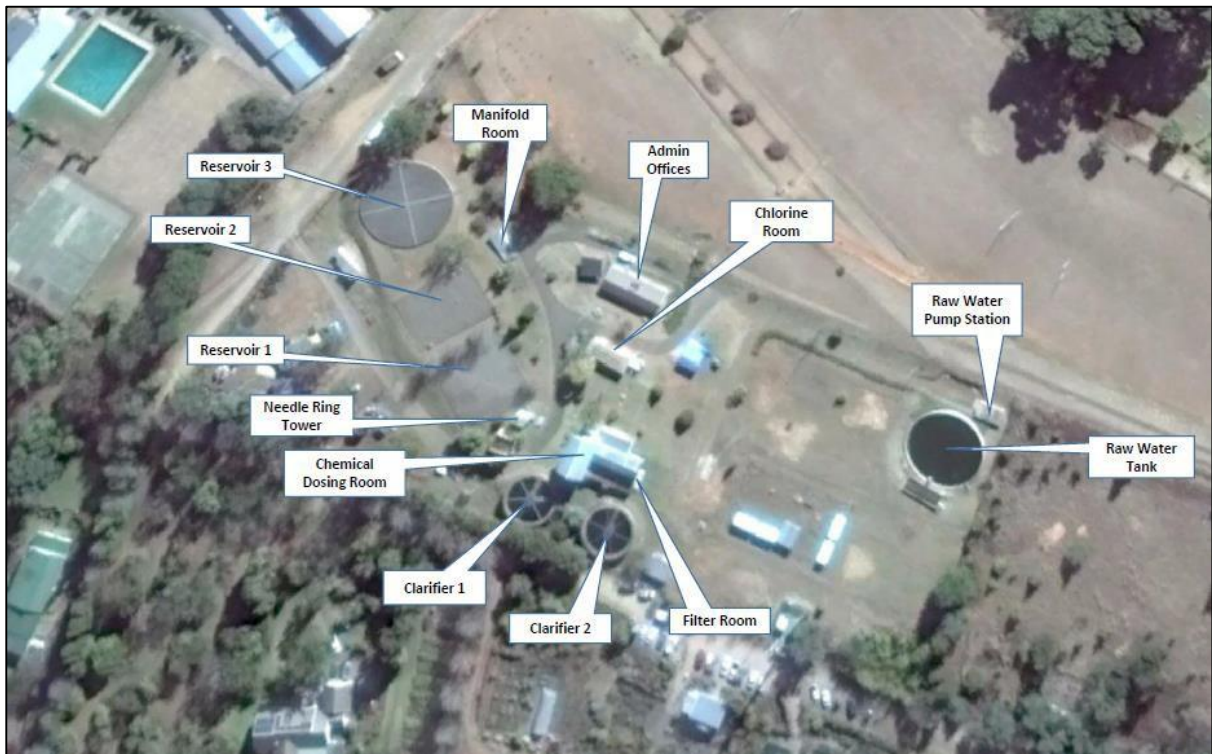
Figure 12.26 Aerial view of the Greytown Water Treatment Plant (Google Earth 2018).
