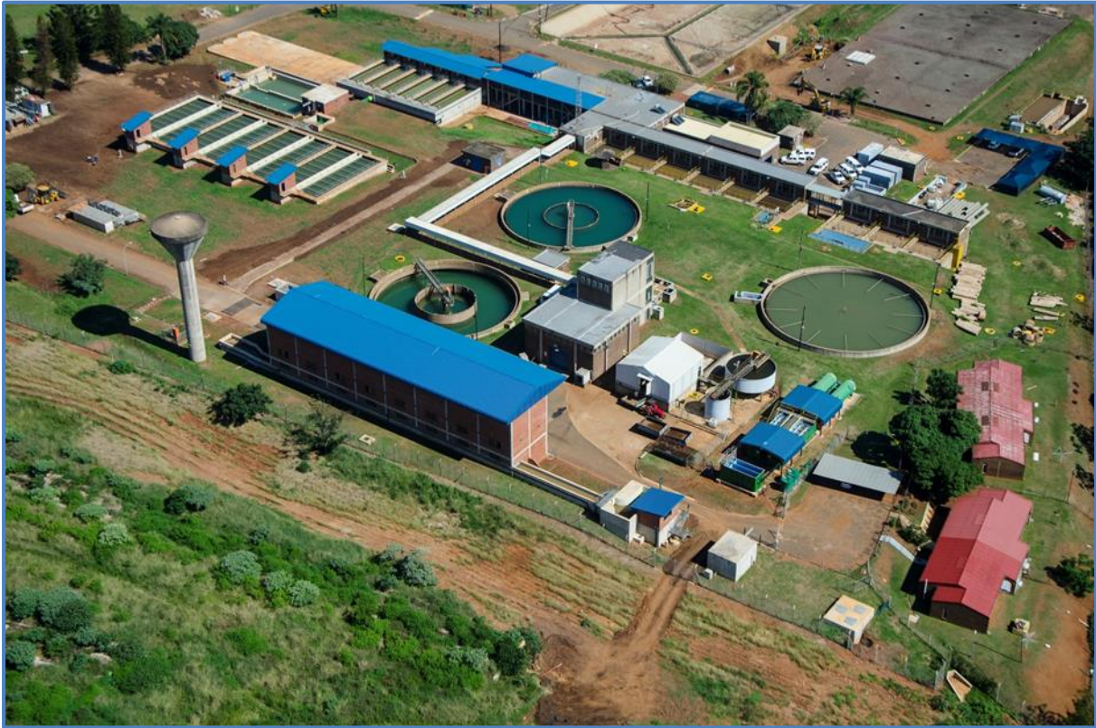
Figure 12.18 Hazelmere Water Treatment Plant.
