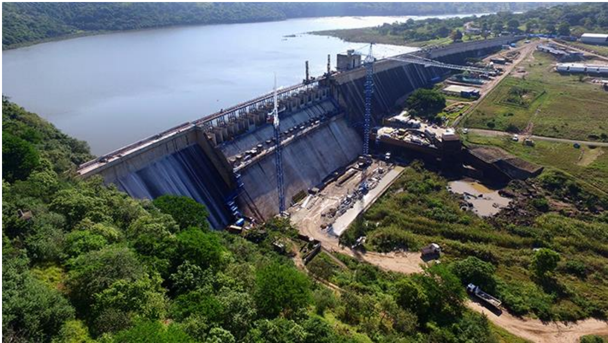
Figure 12.15 Hazelmere Dam showing construction to raise dam wall.
