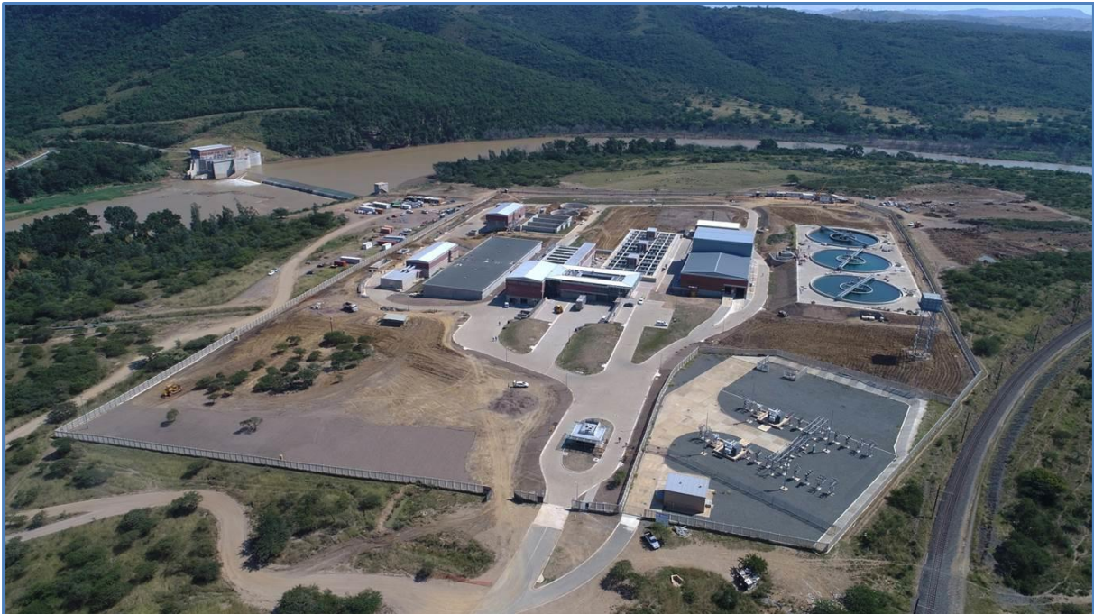
Figure 12.20 Lower Thukela Water Treatment Plant
