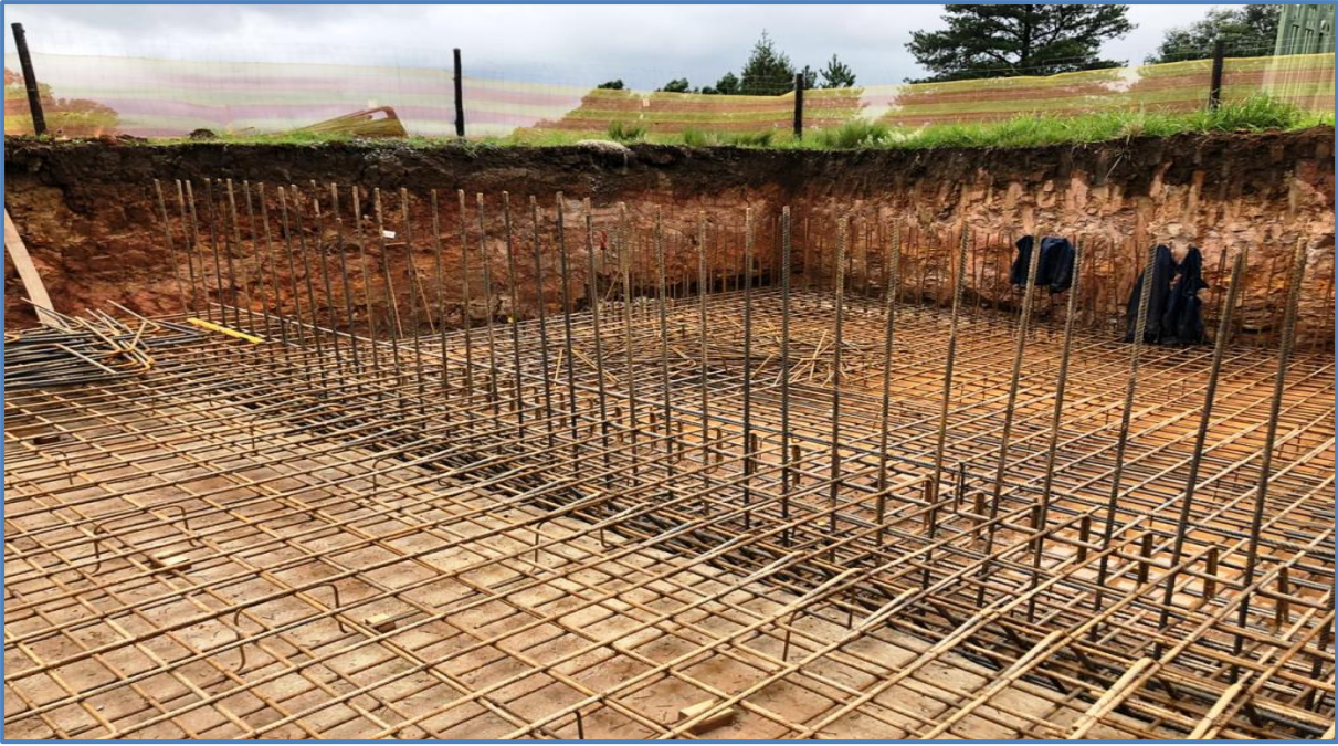
Figure.12.48 Transfer Pump Station in Construction (Late 2019)
