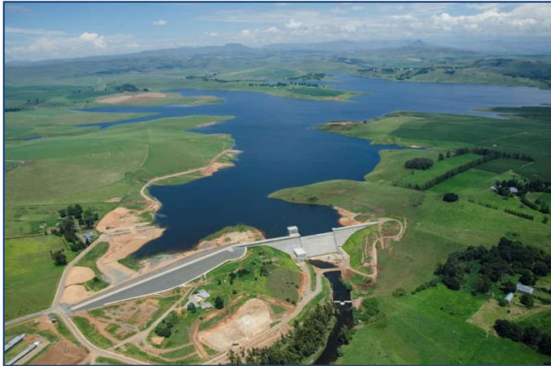
Figure 7.29 Spring Grove Dam.
