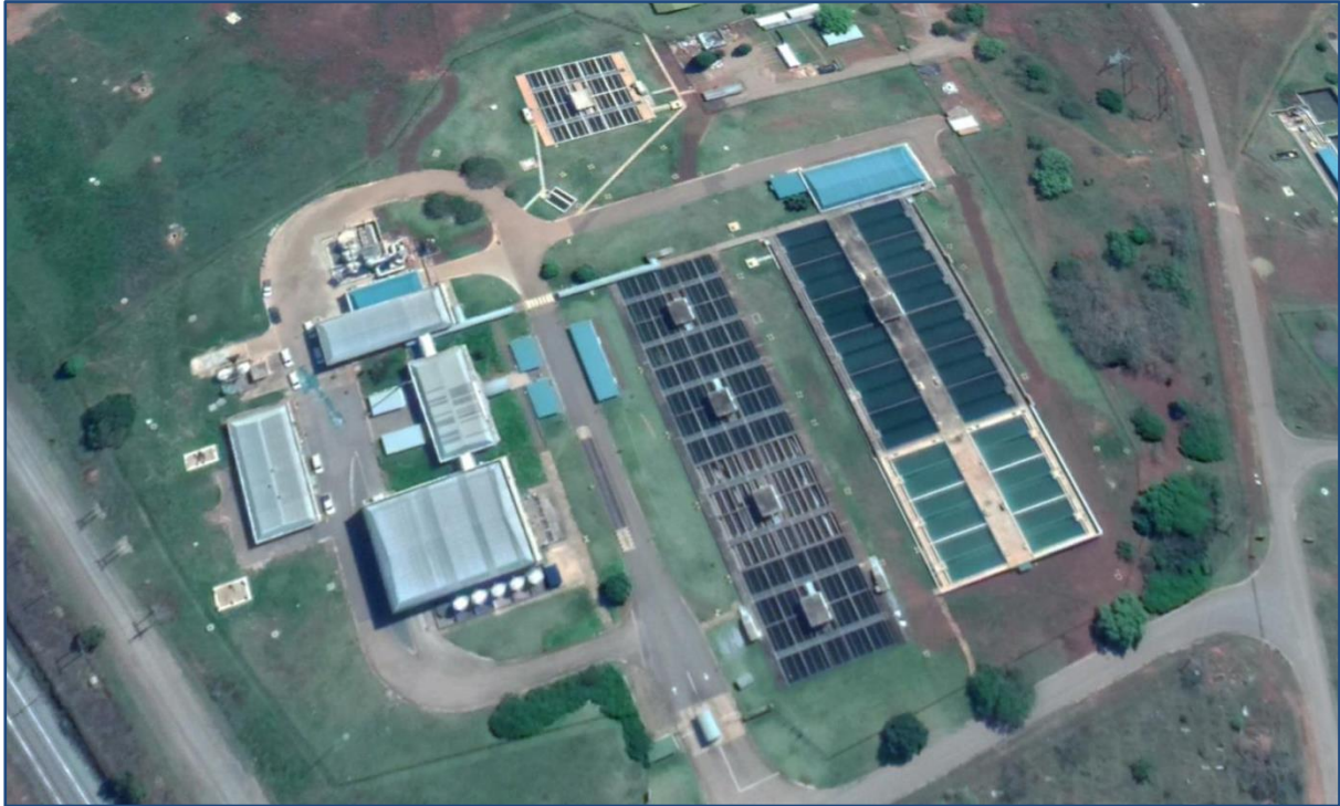
Figure 7.32 Midmar Water Treatment Plant after the upgrade.
