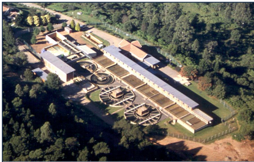
Figure 7.38 D.V. Harris Water Treatment Plant.
