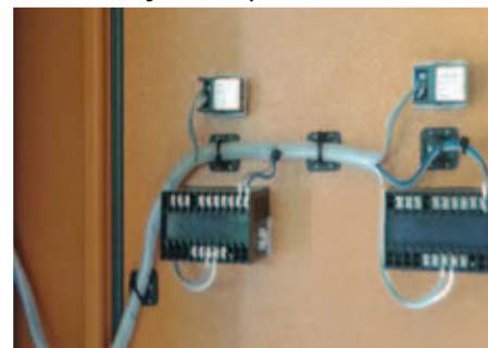
The wiring workmanship by the team
