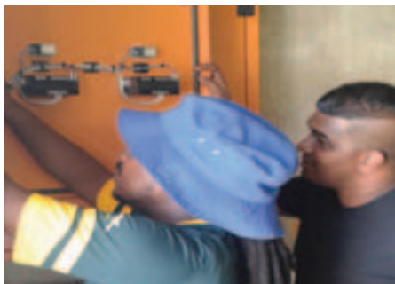
Installing and wiring of new equipment
