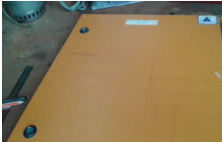
Existing junction box removed for installation of new counters and displays
